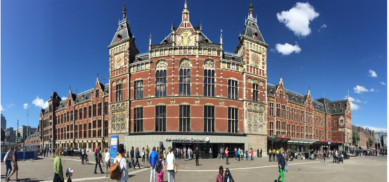
Amsterdam Central Train Station, ©2016 Scott Saier
